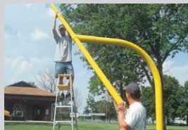
Tip Crossbar to Level and Clamp
