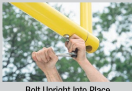
Bolt Upright Into Place
